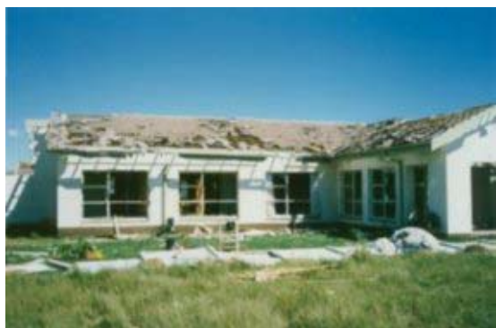
Figure 3. Damage to tiles and glazing.
